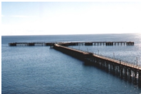
Rapid Bay Jetty. Photo: Jeremy Gramp.
